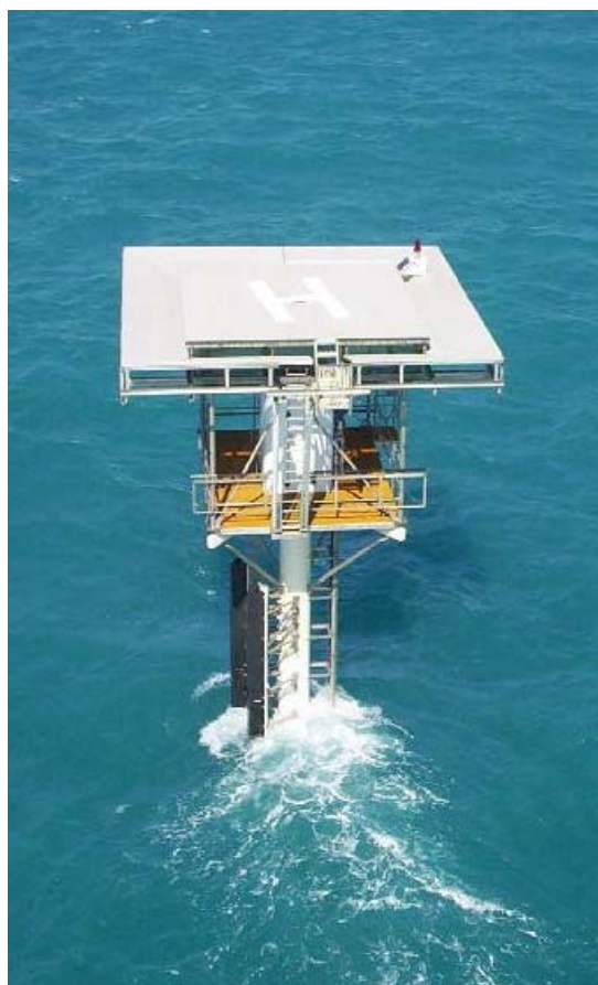
Figure 1. New structure at Nardana Patches
