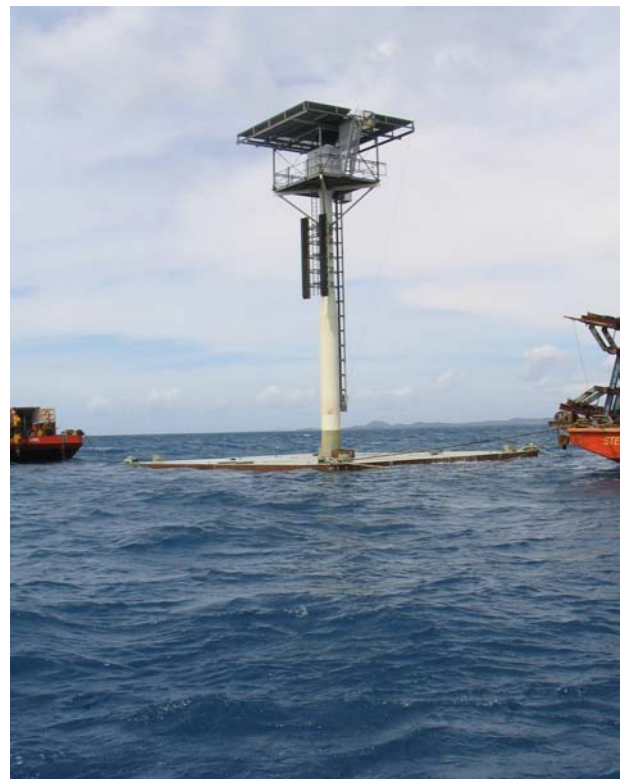
Figure 2. New navaid being installed at Nardana Patches
