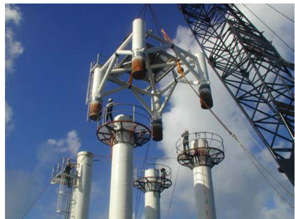
Figure 3. Installing new navaid at Robin Reef
